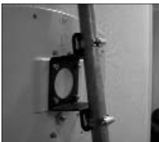
Pipe Mount with Hose Clamp
