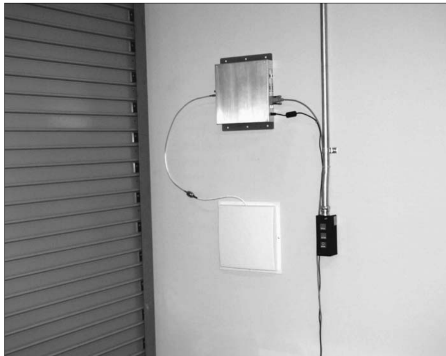
Nanoscanner system configured for a single-antenna portal application. Shown here at a loading dock.
