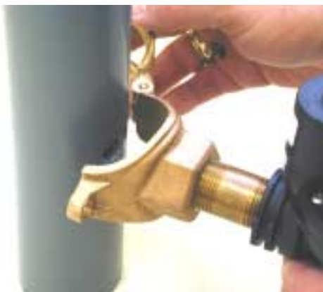
Figure 2-9. Attaching Solenoid Valve Assembly
