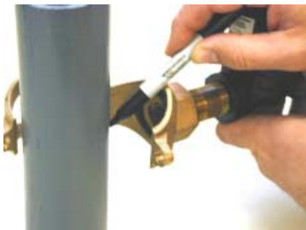
Figure 2-6. Marking Pipe
