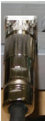
Figure 14: Power Cable Attached
