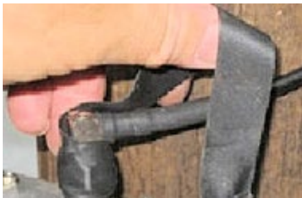
Figure 11: Weather-proof the Connection
