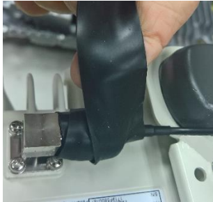
Figure 9: Weather-proof the GPS Connection
