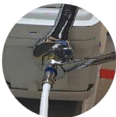
Figure 13: Use 2 Wrenches to Loosen
