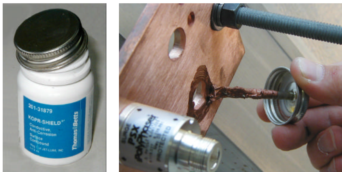
Figure 14: Applying anti-oxidant joint compound
