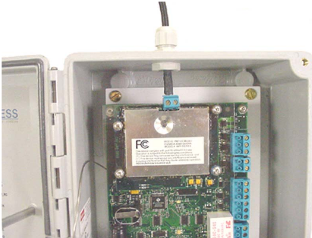
Figure 5-19 – Installing the RAM Coax in the WRI
