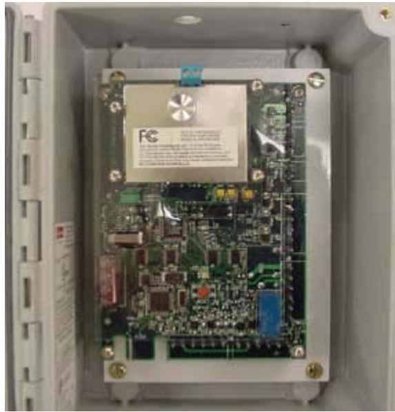
Figure 5-17 – Replacing the WRI's PCB
