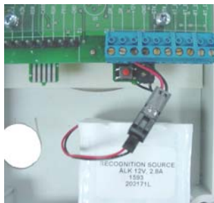
Figure 9-5 – New Battery Pack Installed
