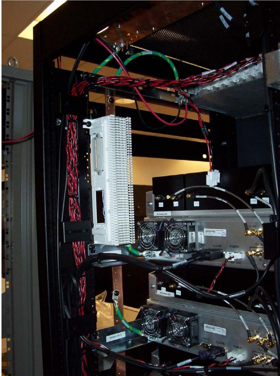
**Figure 25** Punch block location within the MC-Series rack.
