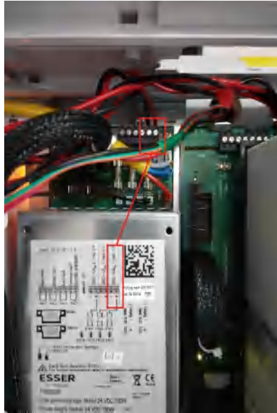
Figure C.8: FlexES Panel Power Connectors
