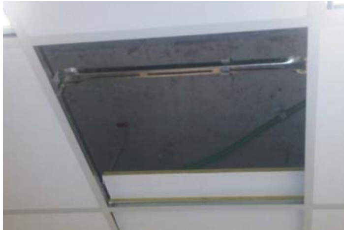
Figure 13: Mounting Clip positioned on a grid of a false ceiling
