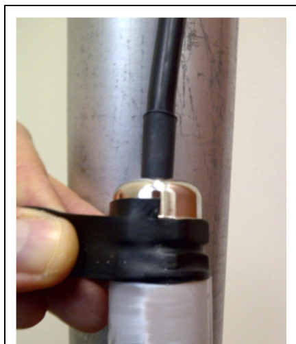
Figure 2-25: Applying sealant tape to an external connection
