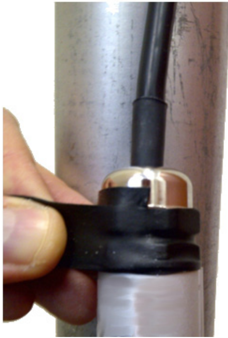
Figure 1-56: Waterproofing an external connection
