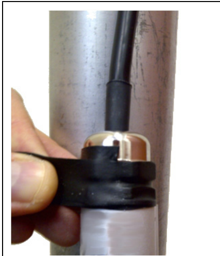
Figure 2-42: Applying sealant tape to an external connection
