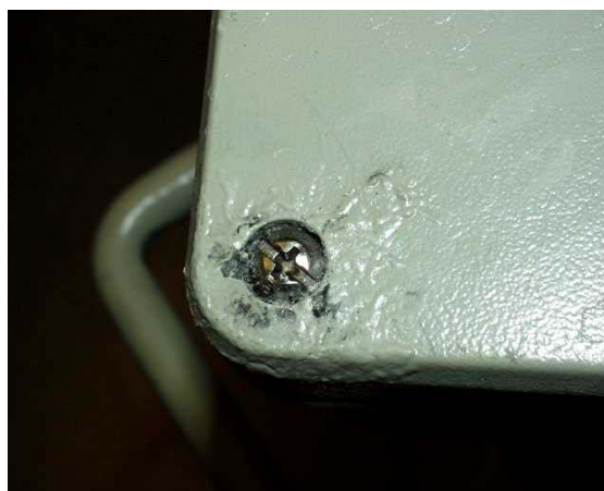
Corrosion attack on Connection box
