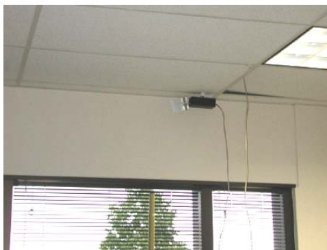
Figure 2. Another typical ceiling mount for PAL-650 Receiver.
