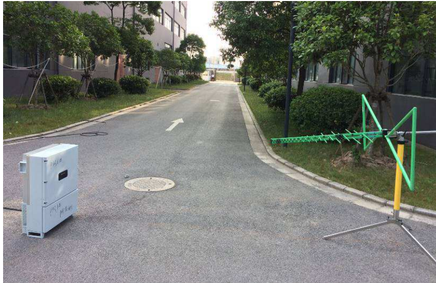
Underground, Location 3, higher than 30MHz
