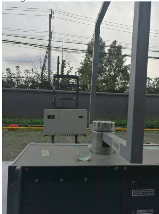
Underground, Location 1, lower than 30MHz
