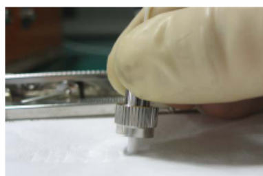
Figure 5-96 Cleaning optical fibers with special cleaning tissues
