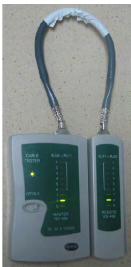
Figure 5-39 Testing the conduction and connections of wires
