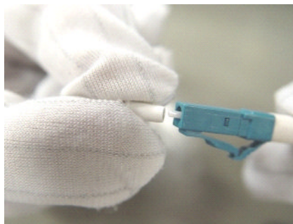
Figure 5-99 Installing a protective cap on a fiber
