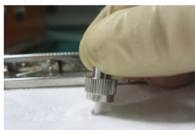
Figure 5-96 Cleaning optical fibers with special cleaning tissues
