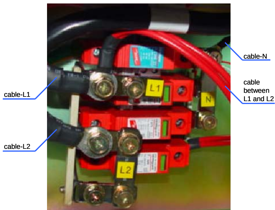
Figure 5-44 Connecting the 110 V power cables
