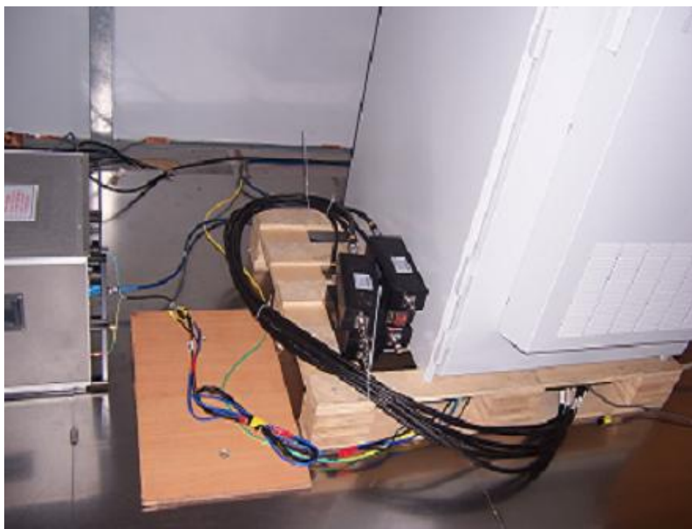
Conducted Disturbance at AC power port
