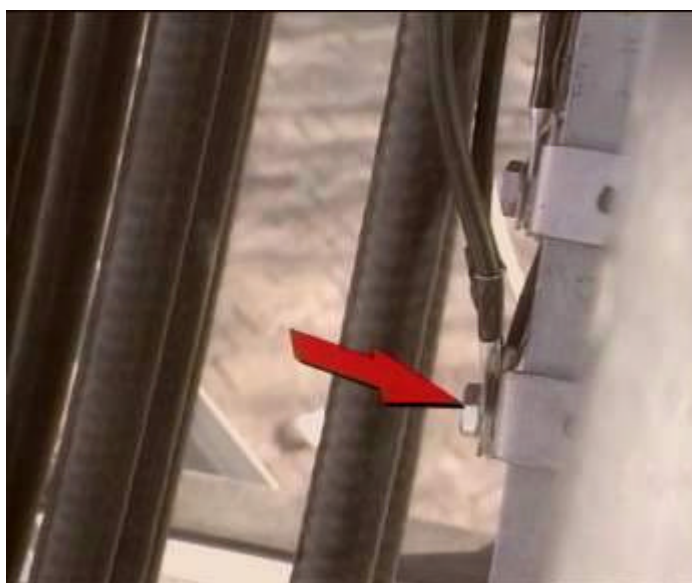
Figure 6-69 Connecting the grounding cable of the feeder grounding clip to the steel plate of the tower
