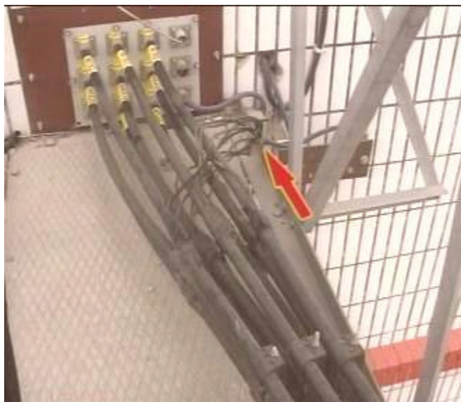
Figure 6-71 Grounding when the feeder does not enter the equipment room (grounding bar unavailable)
