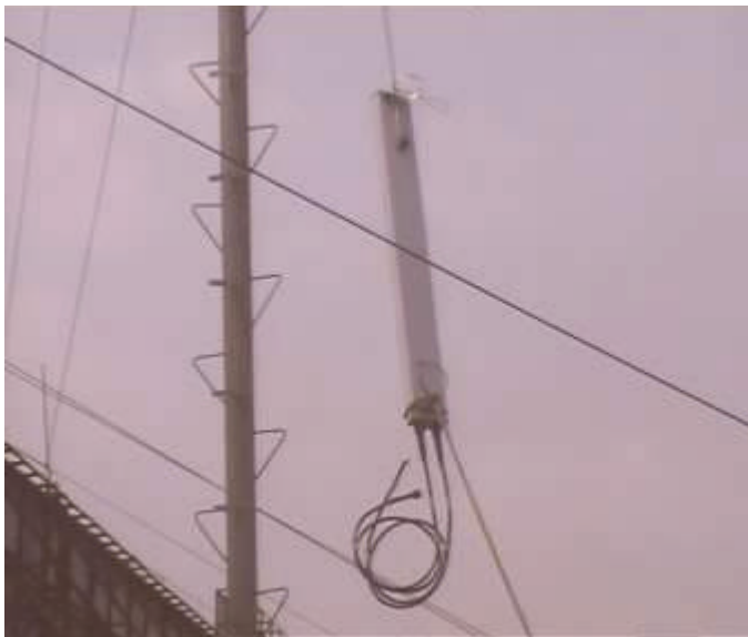
Figure 6-25 Hoisting the directional antenna
