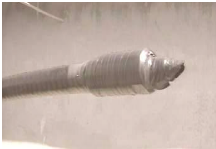
Figure 6-6 Simple waterproof treatment of a connector
