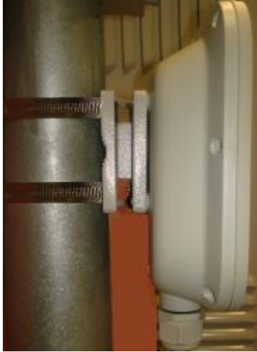
Figure 3-6 Installing the eA360 on the wall-mounting frame
