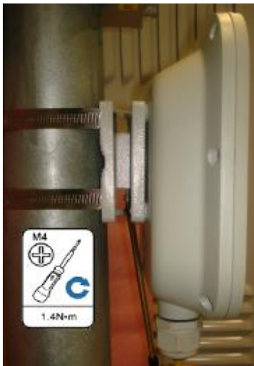
Figure 3-7 Tightening the screw
