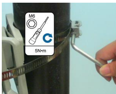
Figure 3-5 Adjusting the length of the hose clamp
