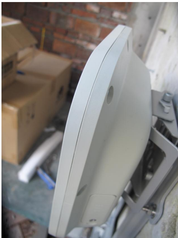
Figure 3-12 Fixing the LTE CPE
