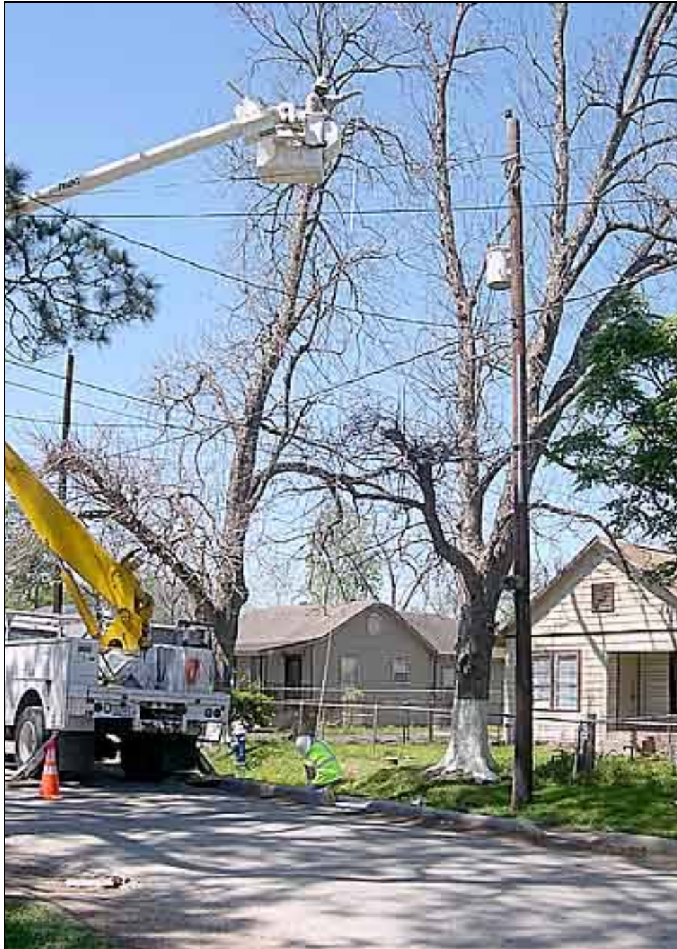
Line Height Measurement
