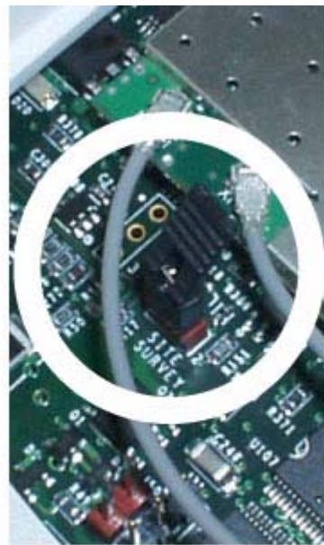
B. Site Survey Jumper Installed
