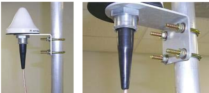
Figure 29 GPS antenna mounting
