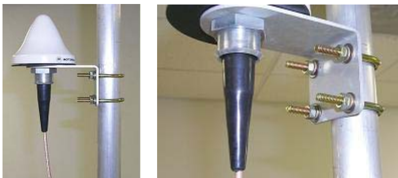
Figure 39 GPS antenna mounting
