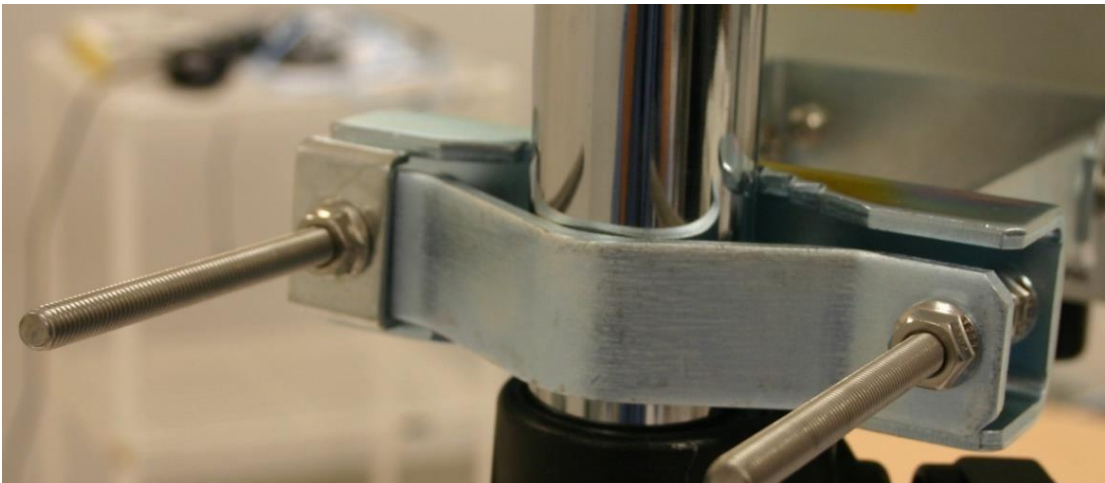
Figure 79 Attaching the AP antenna lower bracket to the pole
