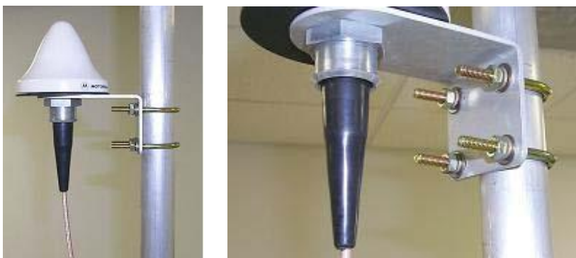
Figure 36 GPS antenna mounting
