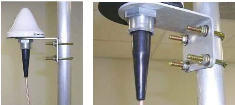
Figure 29 GPS antenna mounting
