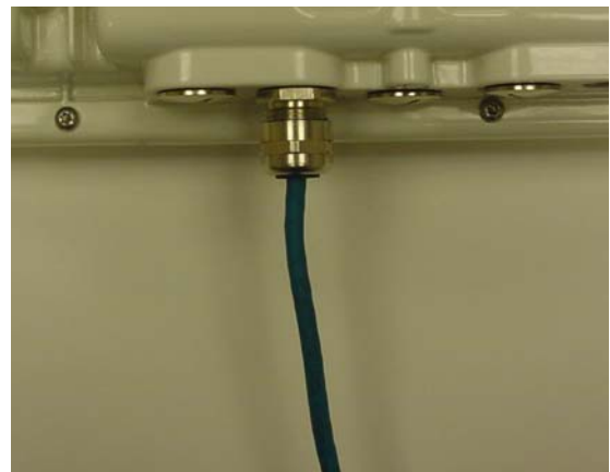
Step 4: Screw on the clamping nut and tighten
