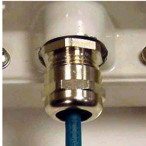
Step 4: Screw on the clamping nut and tighten
