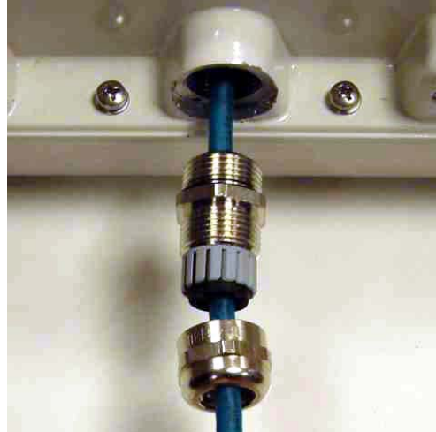
Step 2: Insert the RJ45 connector making sure that the locking tab snaps home
