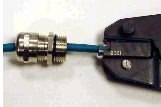
Step 4: Insert conductors and crimp
