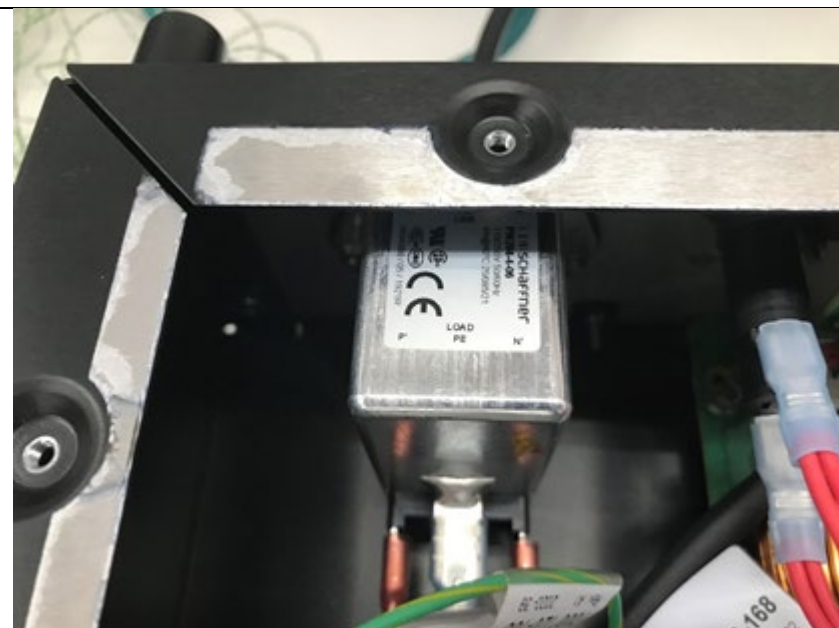
Figure 9: Line Filter View
