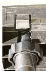
Figure 2.4 Threading the antenna nut
