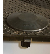
Figure 2.3 Antenna hole in pit lid
