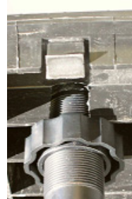
Figure 2.27 Threading the mounting nut
