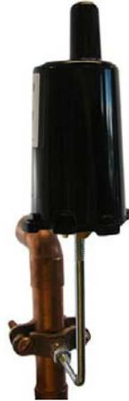
5. Tighten the nut on the mounting rod securely against the pipe clamp to eliminate MLOG sensor rotation.
