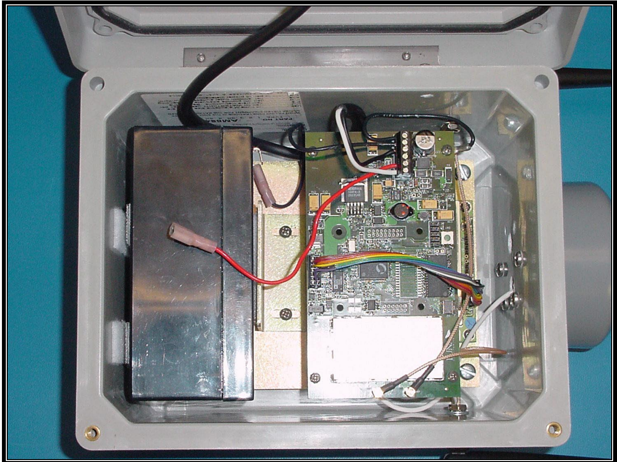
PHOTOGRAPH 6: VIEW INTO ENCLOSURE
