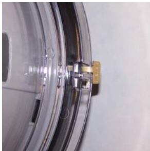
Figure 10 – T-Seal Installed
