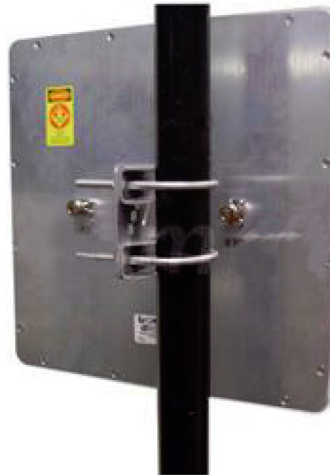
Figure 30. Installing Flat Panel Antenna to the Pole
