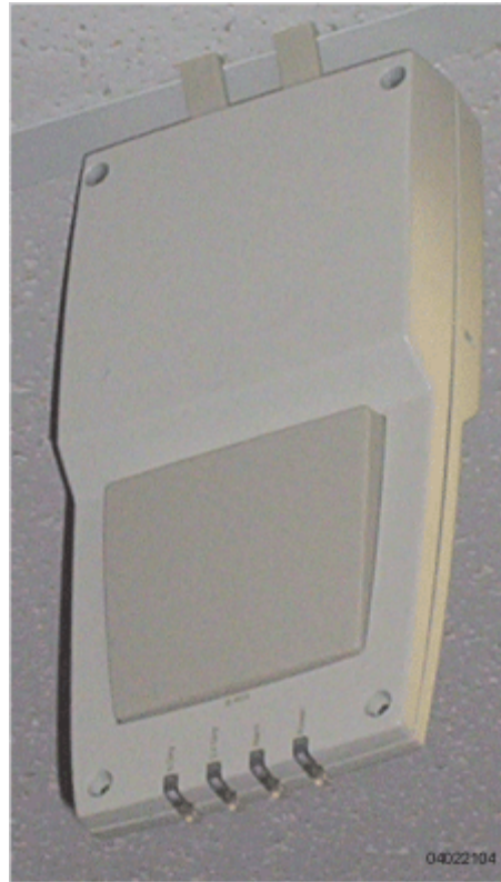
Figure - Clipping the OmniAccess AP and Ceiling-Mount Clips to a Hanging-Ceiling Rail
