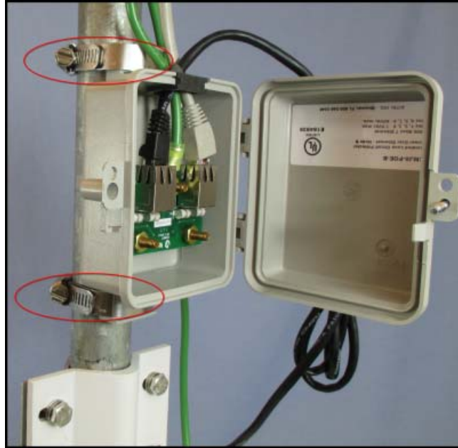
Figure 8 Hose clamps to mount Citel surge suppressor
