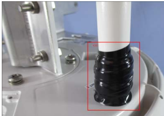
Figure 29 Outer layer of tape on antenna connection
