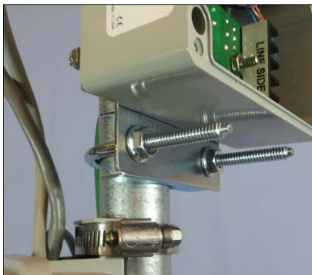
Figure 17 L-com serial surge suppressor mounted with a U-bolt
