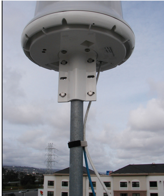
Figure 2-9 Secure Ethernet Cable
