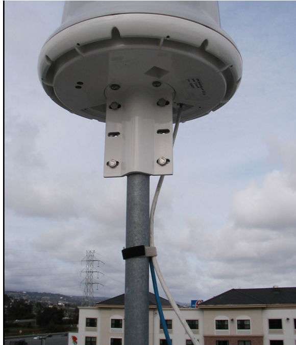
Figure 2-13 Secure Ethernet Cable
