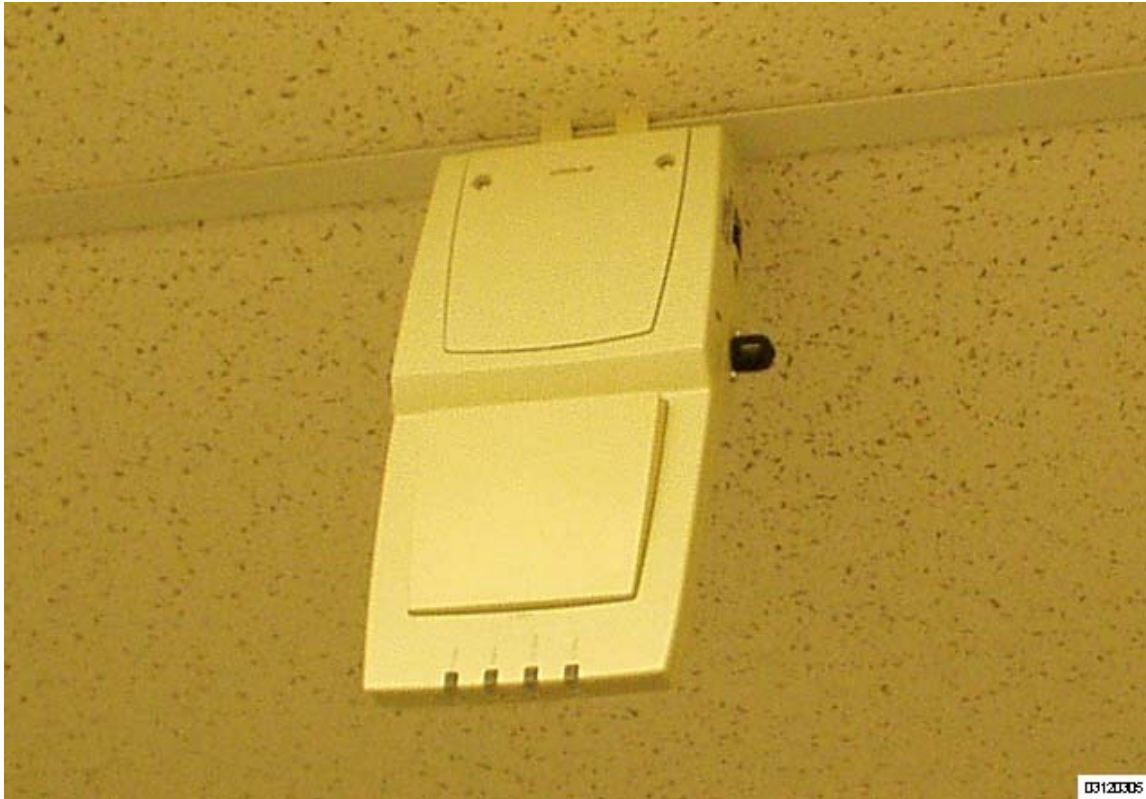
Figure - Clipping the Nortel Networks WLAN - Access Point and Ceiling-Mount Clips to a Hanging-Ceiling Rail
