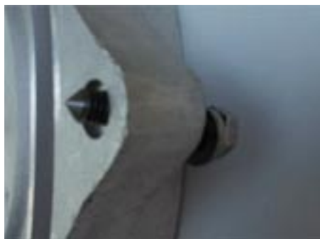
Figure 3-9.1 Captive radio bolt detail
