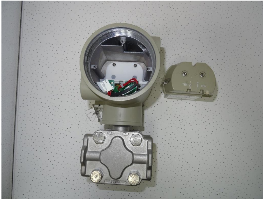
Photo 5: Host battery removed
