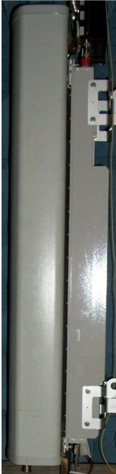
RRH 2x45W 1900MHz RF151032 with antenna assembly
