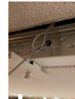
FIGURE 3 Attaching the Cable to a Structurally Sound Anchor
